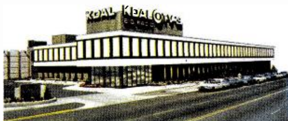
KDAL BROADCAST CENTER COMPLETED IN 1968
